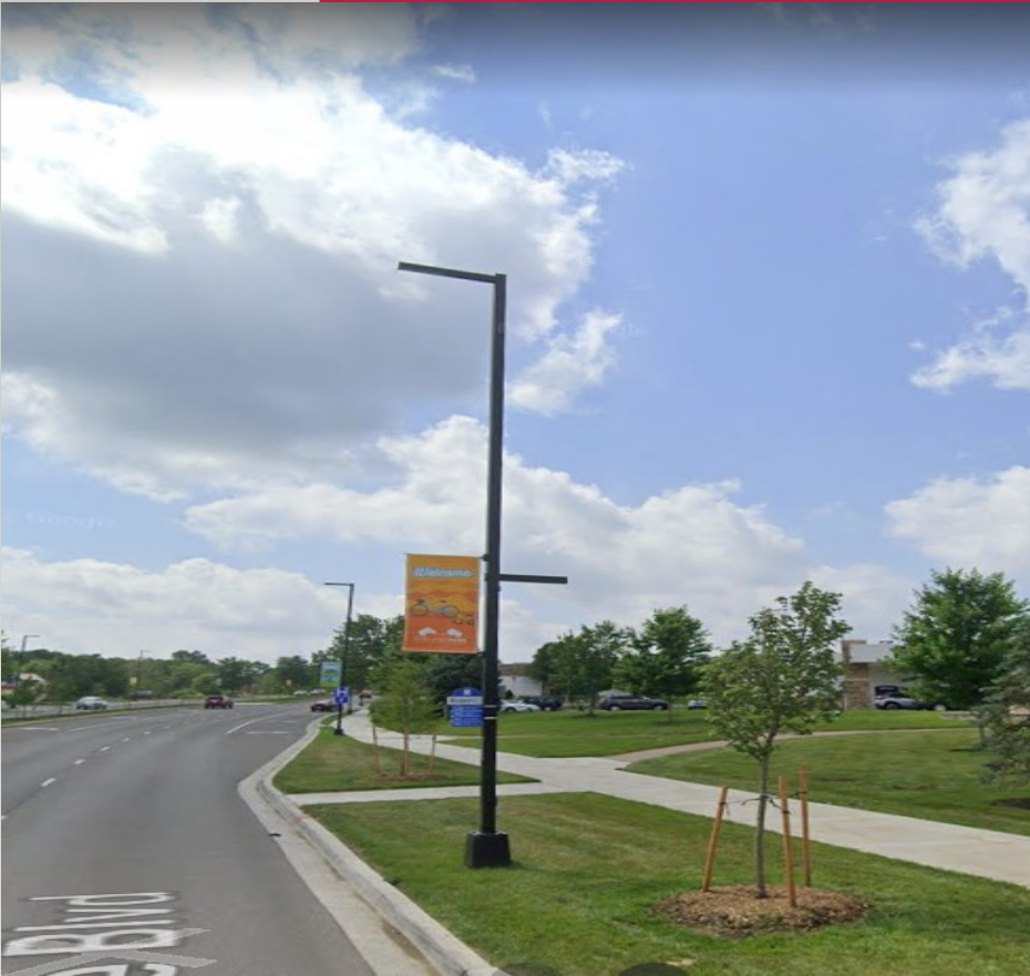
Roe Blvd Streetlighting – 30' pole with 14' pedestrian light
