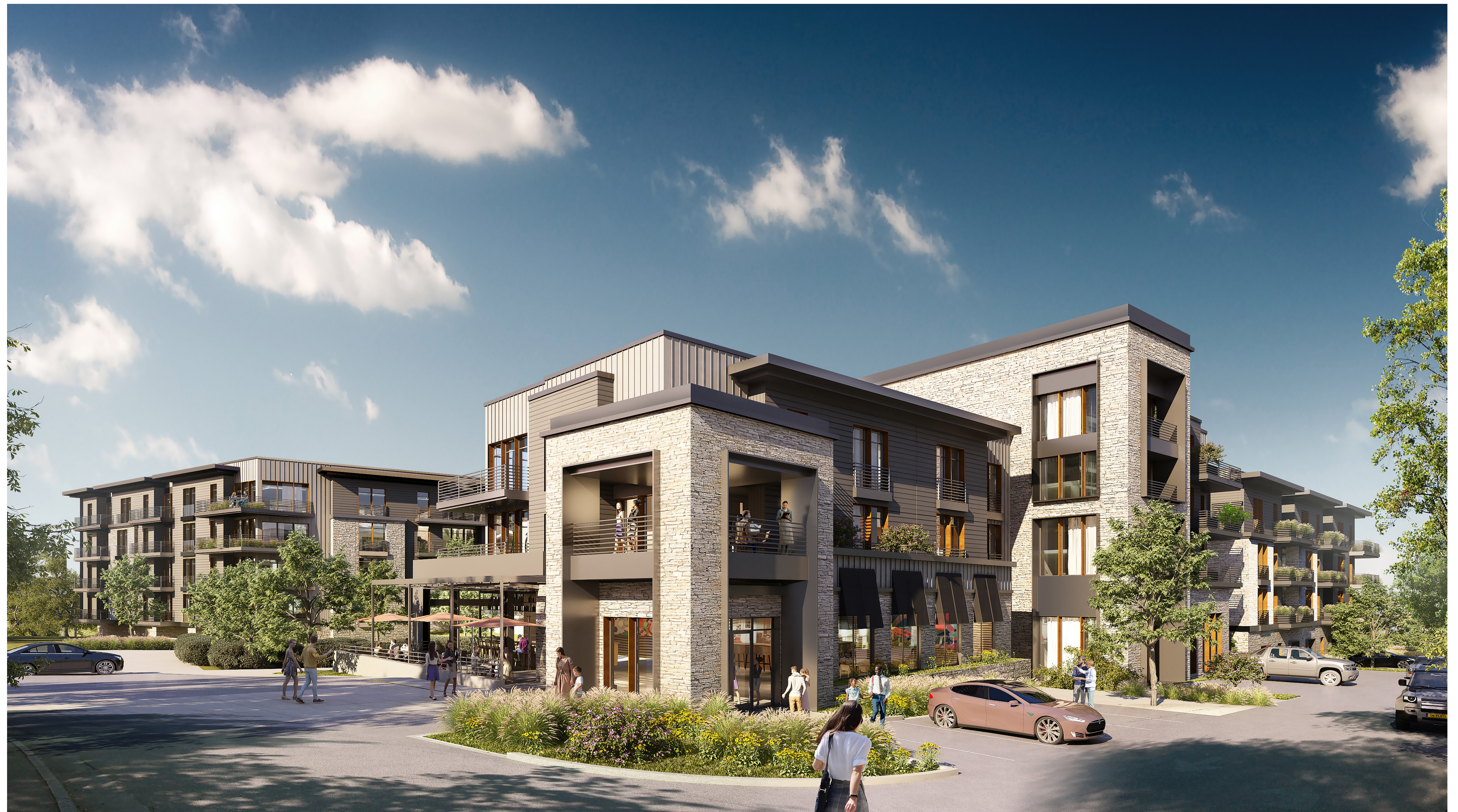
VIEW OF COMMERCIAL SPACE FROM NORTHWEST VEHICULAR ACCESS
